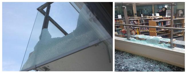
4. On balustrading systems, friction only glass clamps are prohibited unless the glass is fully supported at its base (and sides on sloping glass panels). Insufficient restraint to glass panels on balustrades can cause the panels to become dislodged or come loose, or in the worst case fall from their original position with obvious consequences.
